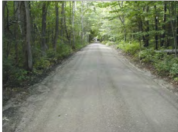
After - Same section of road with new surface gravel, crowning, and grader berms removed.
