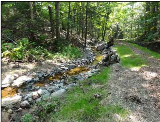
After - Lower reach stabilized with pool and cascade structures, riffles, and rock veins.
