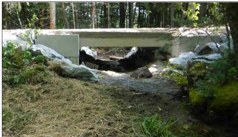
The Fitts Mountain Road stream crossing in Dedham was replaced with combined funding from a Stream Crossing Grant ($20,000) and CWA Section 319 ($8,665) as part of Hancock County SWCD’s Phillips Lake Watershed Protection Phase II Project.
